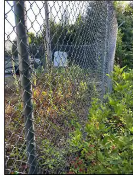
Photo 6: Top of slope at southeast corner of Survey Area / fence, facing southeast.
