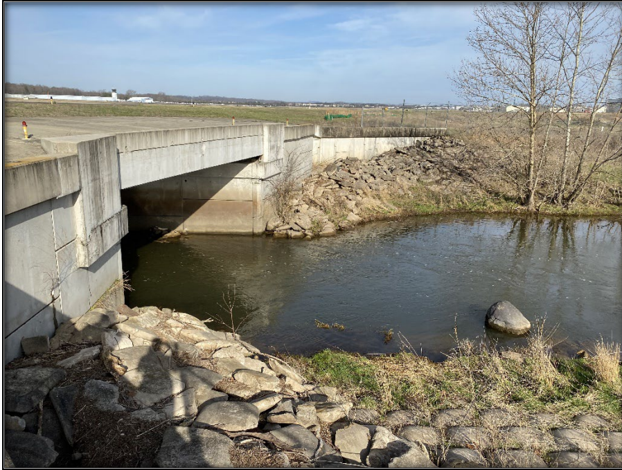
Photograph 5. View of Broad Run flowing beneath the airport runway.
