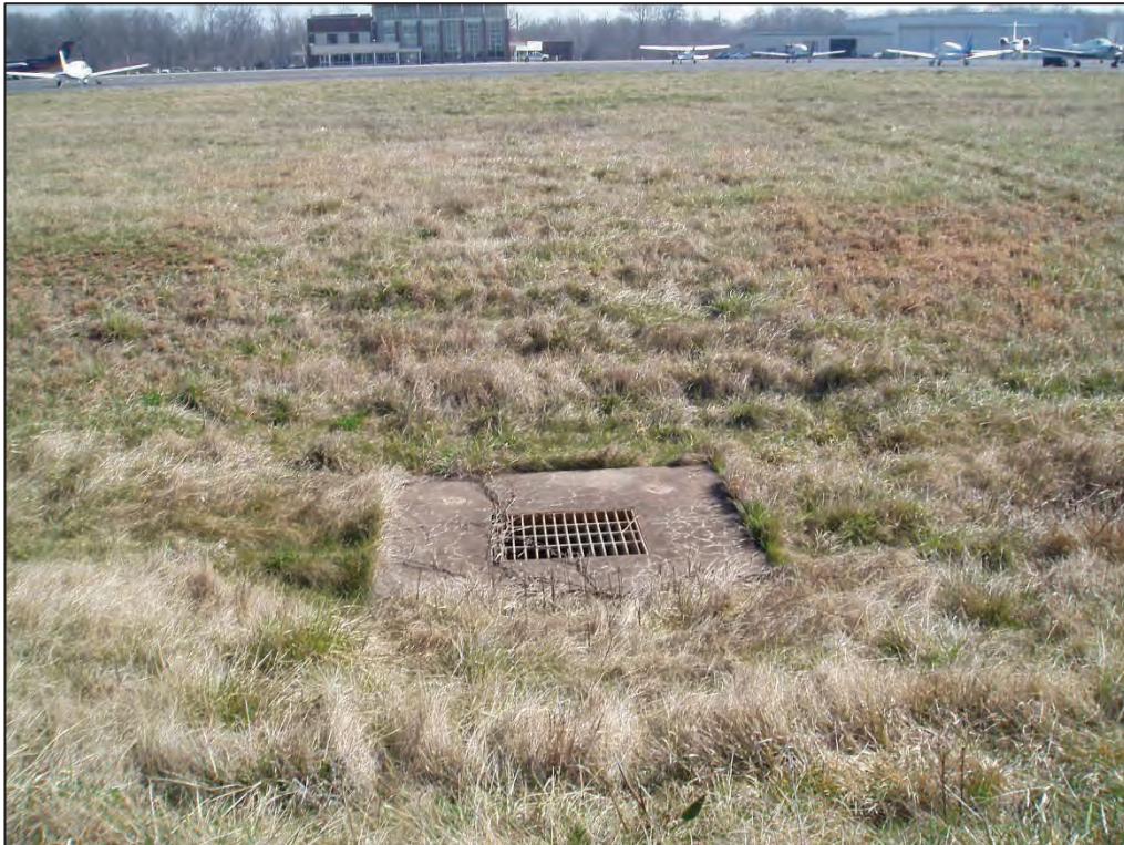
Photograph 22. Looking E across the grassed infield area that will hold proposed Project #9. The existing terminal's west façade is in the background (Field Photograph CSW_P3140025, 03/14/2024).
