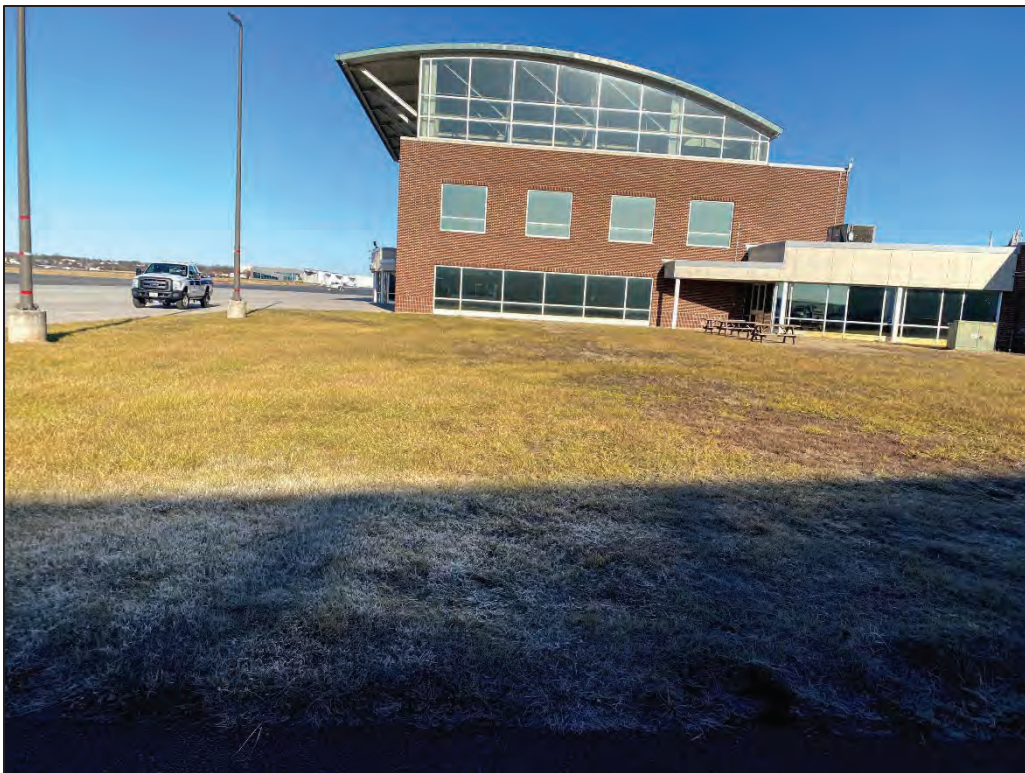
Photograph 4. Looking N at the south façade of the existing HEF Terminal. The east side of the Phase 1 L-shaped terminal extension will be located in this grassed area (Field Photograph JM_IMG8757, 01/11/2024).
