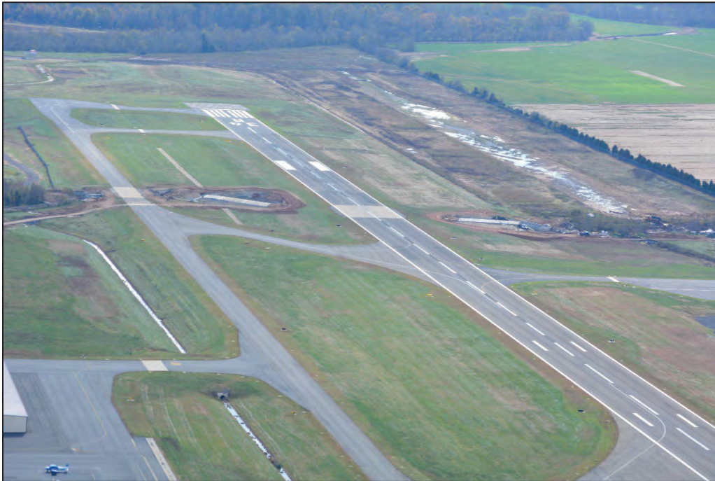
Photograph 15. Looking SW at T/W B (left) and R/W 16L/34R (right) during the bridge replacements in 2014. The by-pass channel is in the photo's upper right (Field Photograph Airport_DSC0563, 2014).
