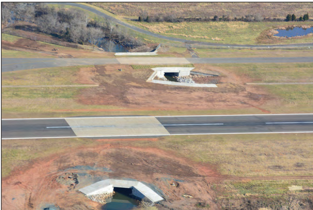
Photograph 16. The new 2014-2015 T/W B and R/W 16L/34R bridge structures (Field Photograph Airport_DSC0191, 2014).
