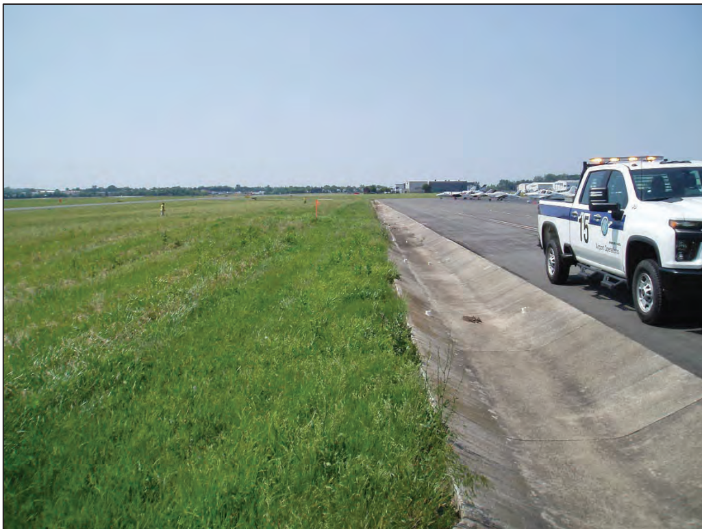
Photograph 8. Looking N at the west edge of the East Ramp and its existing drain. The bioswale as depicted on the concept includes part of the grassed area to the west.
