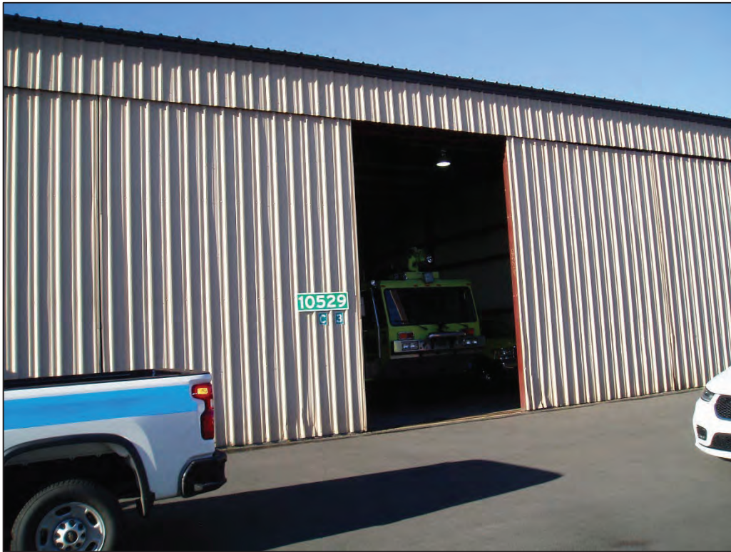
Photograph 23. Looking at the east façade of T-hanger building 10529 that currently hosts the Airport's fire trucks (Field Photograph CSW_P1110002, 01/11/2024).
