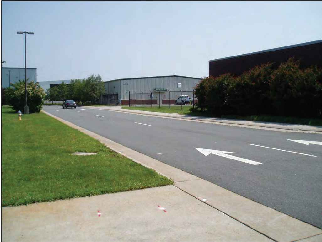
Photograph 9. Looking SW at the existing terminal parking lot loop (Field Photograph CSW_060525).
