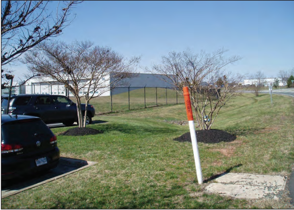
Photograph 21. Looking NW at the proposed SRE building lot (beyond fence). The Wakeman Drive ROW hosts a buried cable, and, behind the cable post, a stormwater structure manhole cover (Field Photograph CSW_P3140040, 3/14/2024).
