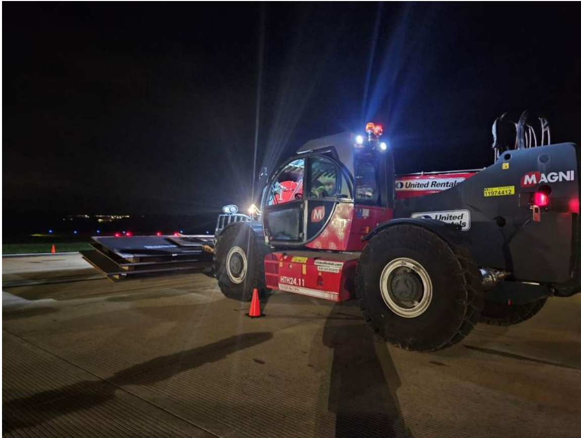
Figure 7. Loaded Forklift on the Runway Bridge.
