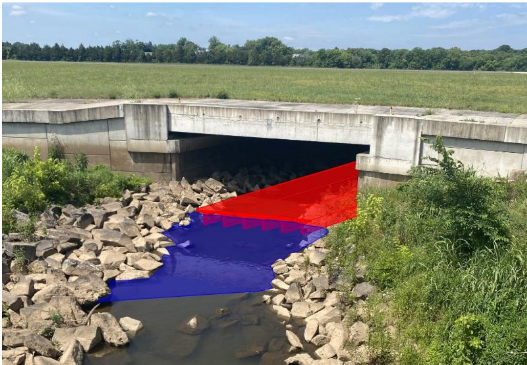
Image #1 – Preliminary Concept – Double-Tees as working surface to maintain stream flow underneath.
