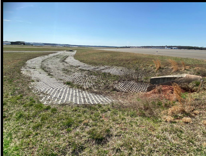
Photograph 11 – View west of infield drainageway north of Wetlands C and D. (03/12/2024)
