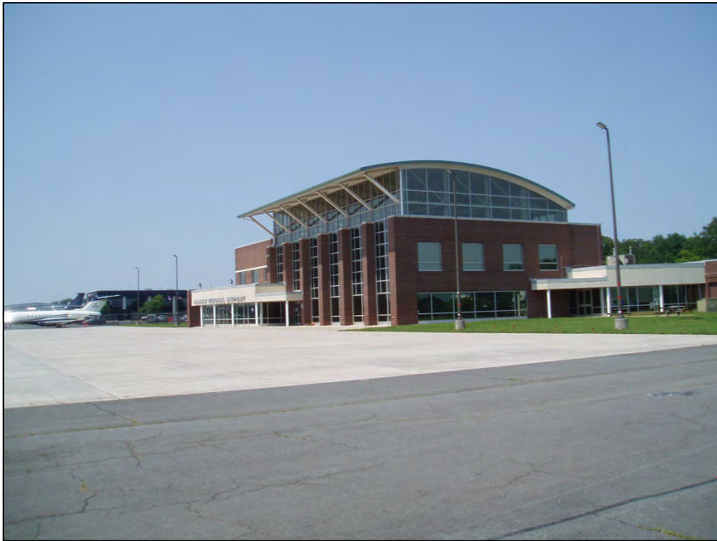
Photograph 3. HEF Terminal, looking NE at the south and west facades (Field Photograph CSW_060425).
