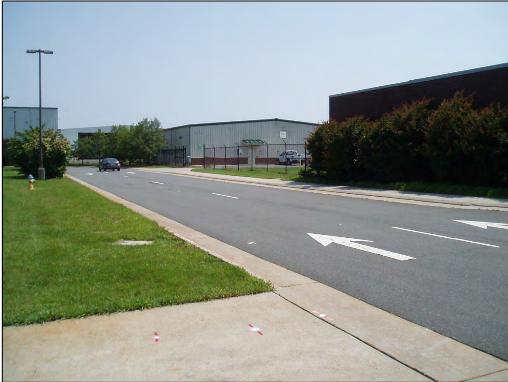
Photograph 9. Looking SW at the existing terminal parking lot loop (Field Photograph CSW_060525).
