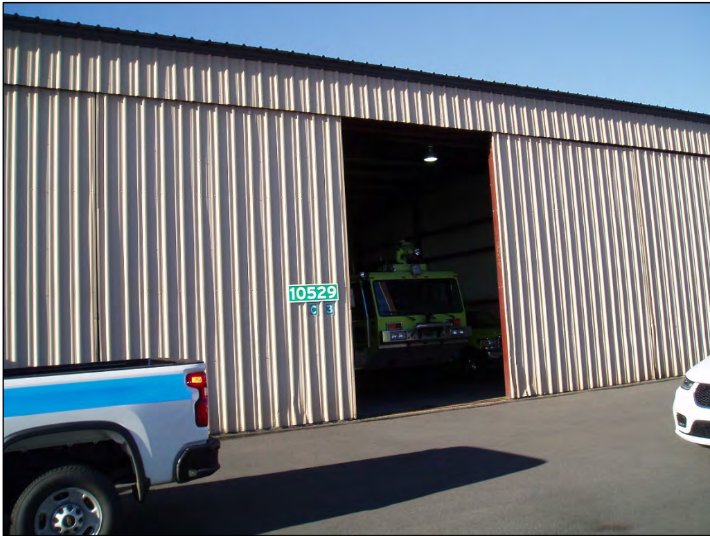
Photograph 23. Looking at the east façade of T-hanger building 10529 that currently hosts the Airport's fire trucks (Field Photograph CSW_P1110002, 01/11/2024).
