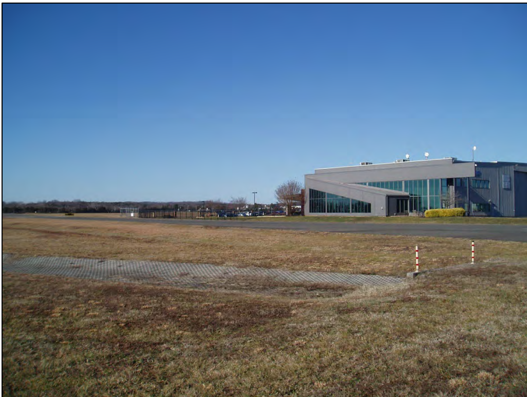
Photograph 24. Proposed location of the New ARFF Building, looking NW (Field Photograph CSW_P1110017, 01/11/24).
