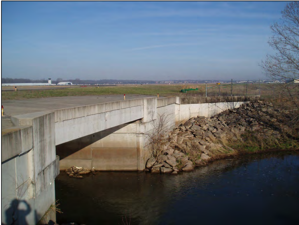
Photograph 17. The existing east side of the Cannon Branch bridge structure underlying T/W B (Field Photograph CSW_P3140005, 03/14/2024).
