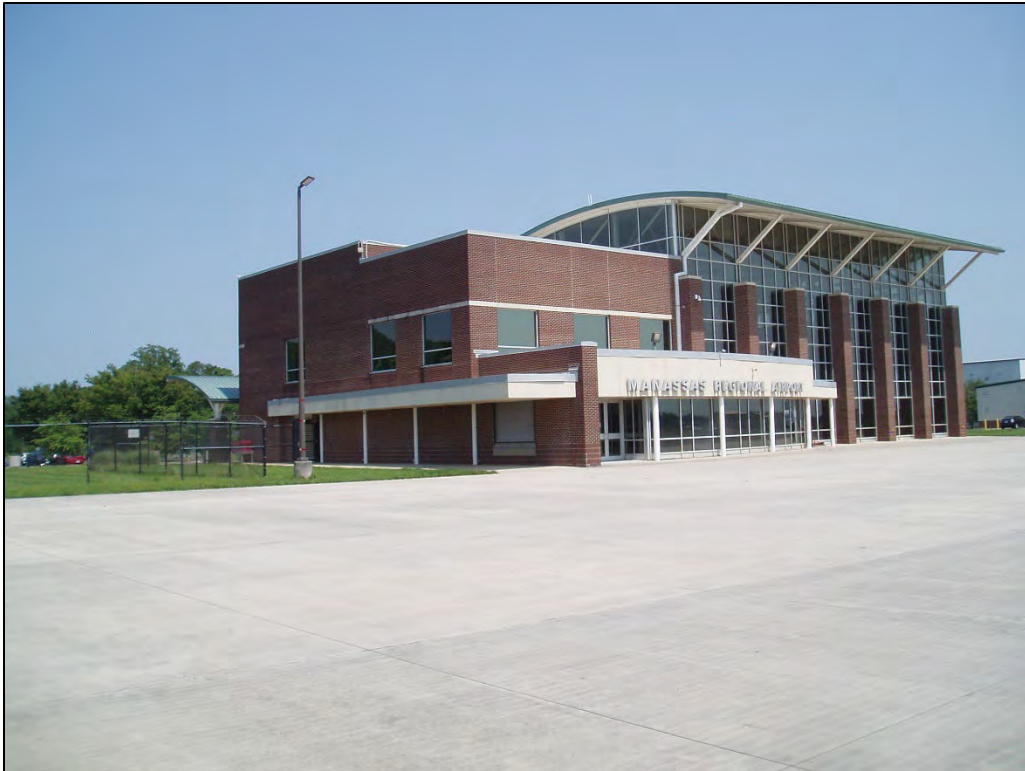
Photograph 1. HEF Terminal, looking SE at the north and west facades (Field Photograph CSW 060425).
