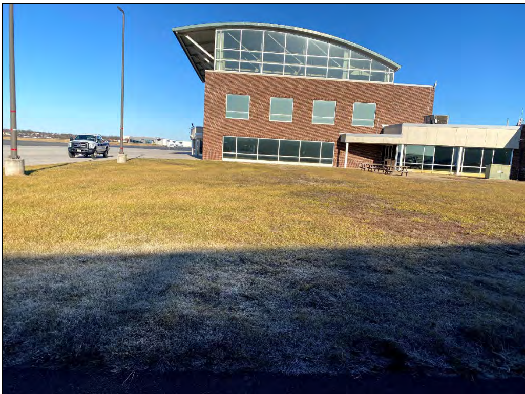
Photograph 4. Looking N at the south façade of the existing HEF Terminal. The east side of the Phase 1 L-shaped terminal extension will be located in this grassed area (Field Photograph JM_IMG8757, 01/11/2024).
