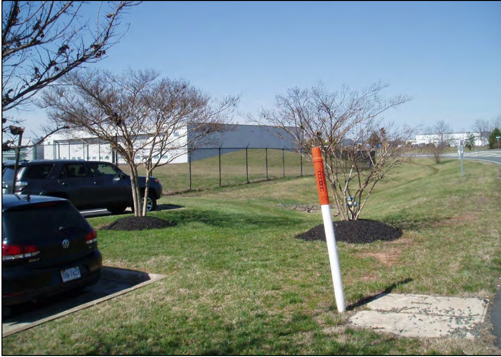
Photograph 21. Looking NW at the proposed SRE building lot (beyond fence). The Wakeman Drive ROW hosts a buried cable, and, behind the cable post, a stormwater structure manhole cover (Field Photograph CSW_P3140040, 3/14/2024).
