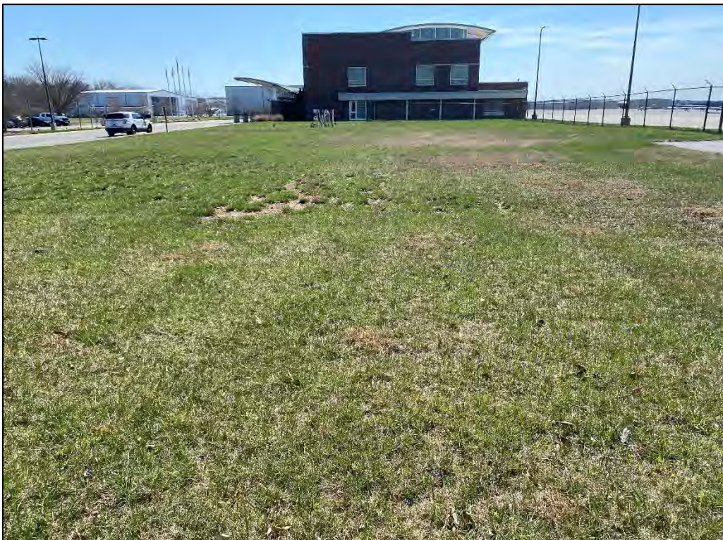
Photograph 2. Looking S at the north façade of the HEF Terminal. The grassed area will host a Phase 2 terminal extension (Field Photograph JM_IMG0462, 01/11/2024).
